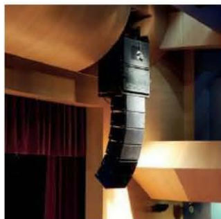
Two powered LX-215RA subwoofers per side are rigged in a cardioid configuration above the Aero 12As
